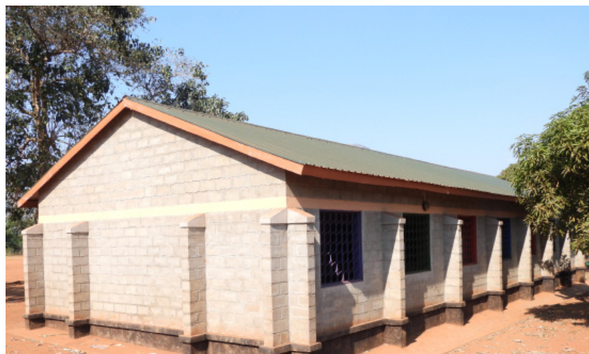
) Newly rehabilitated classroom block at Muloza Primary School in Mulanje. Pictures by Robert Nayeja. MANA.
