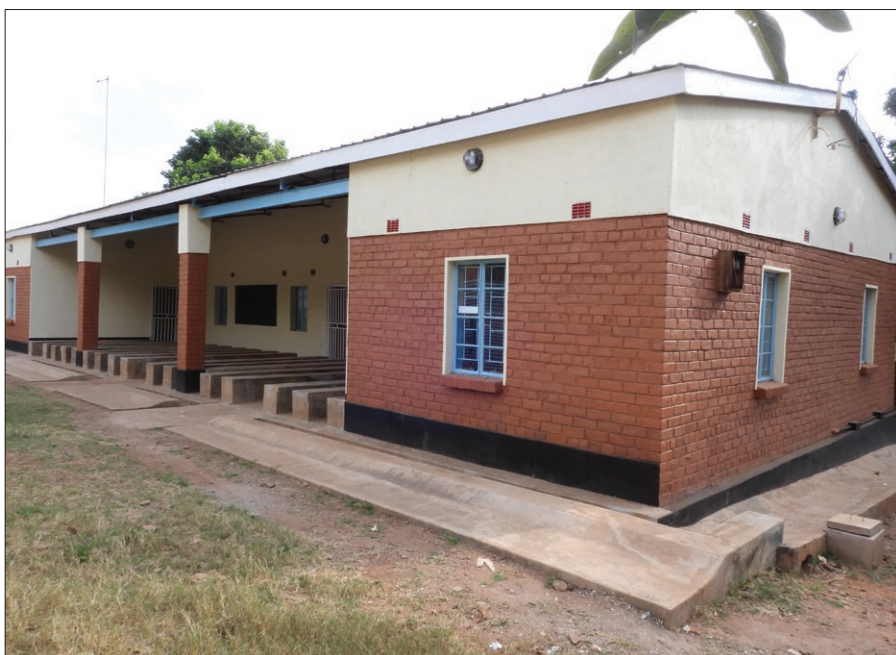
The renovated maternity wing at Chambe Health Centre.
