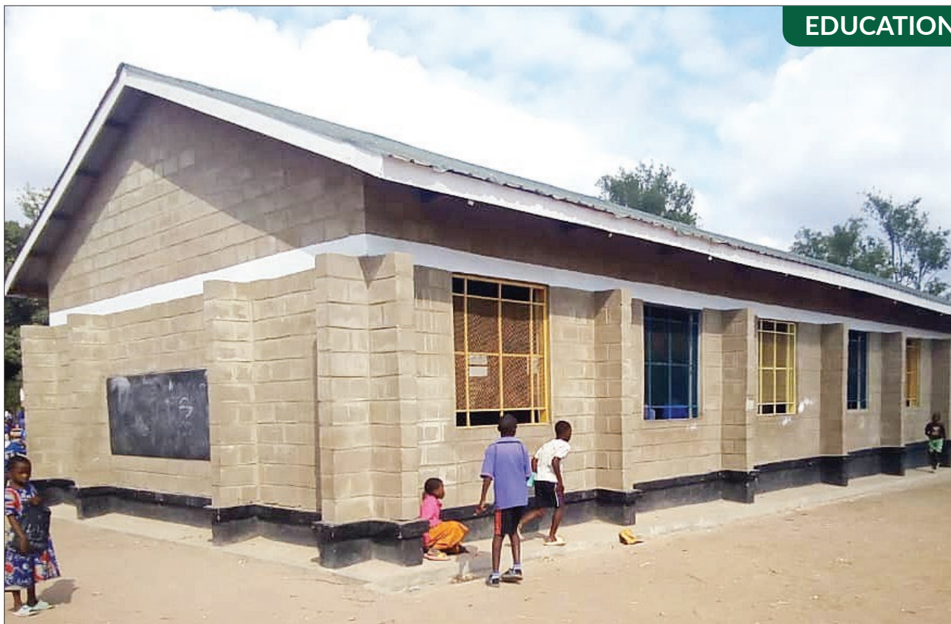
The new classroom block at Ngokwe Primary School in Machinga.
